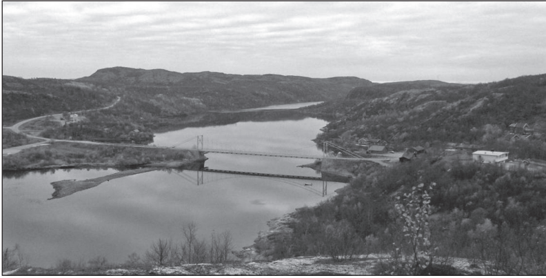
Figure 2. The Pasvik River bridge at Elvenes.
